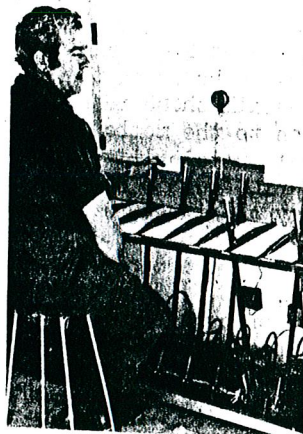
A.M.S.R.S. SIGNAL BOX
